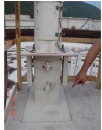
Left to right: 1) 6" UNI Flange, 2) Centering of stilling well 3) Good example. Stilling well can move vertically free from the platform. 4) Bad example. Stilling well is fixed to the platform.
