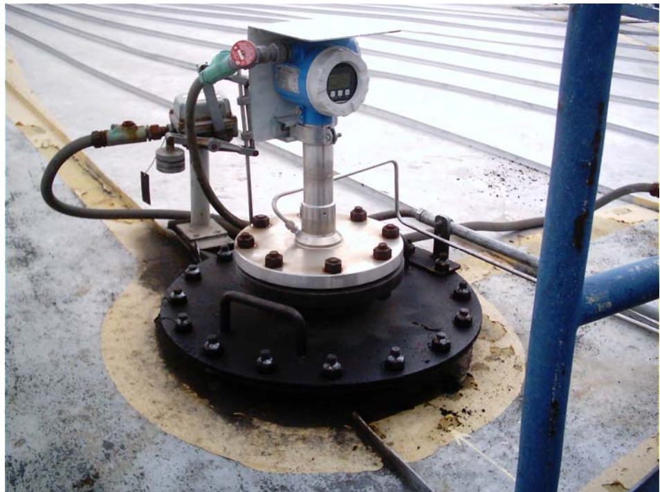
7230 Radar Tank Gauge with large horn, low frequency, high temperature and air purge options
