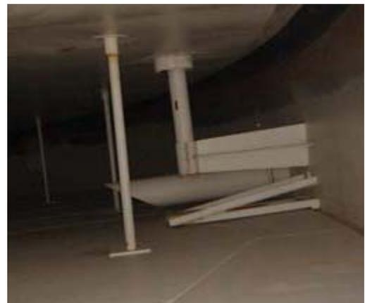
For tank floor support, a simple tripod is sufficient. For tank shell support, it is important that a certain amount of tank 'bulging' (due to hydrostatic tank deformation) can be tolerated without extreme mechanical stress exerted on the tank shell itself.
