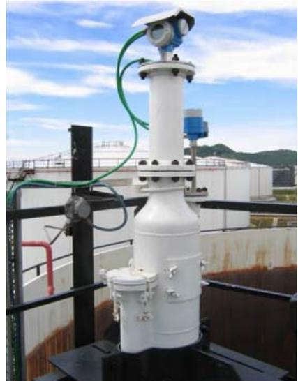
It is advised to make the whole stilling well the same diameter, especially in the case when a radar level gauge is used. Changes in pipe diameter change the speed of radar and, thus, the absolute accuracy of a system. This is less critical with other gauge technologies, such as servo gauges.
