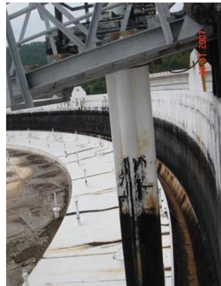
Note: It is assumed that the top of the stilling well is ‘open’ and not hermetically sealed. The opening can be inside the tank and below the roof provided the highest hole or perforation is well above the maximum safe oil level for the tank. Failure to follow these guidelines can lead to serious level errors and, in worst case situations, even to overfills and product spillage.
